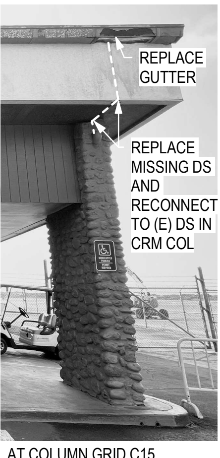
AT COLUMN GRID C15
