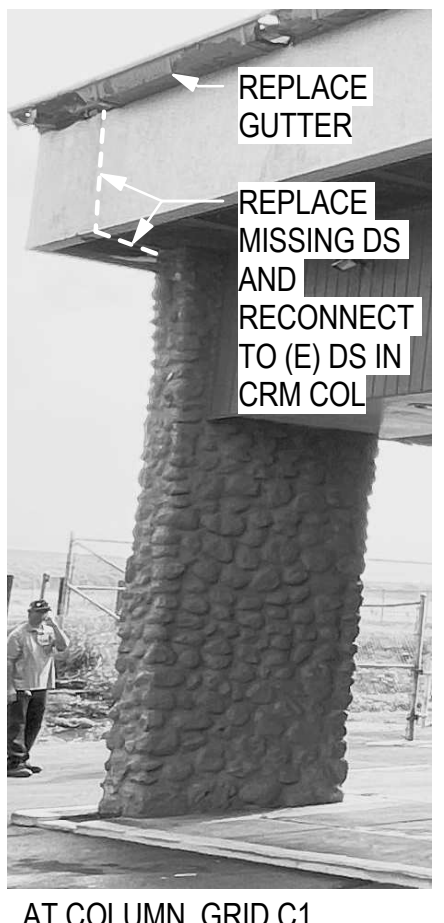
AT COLUMN GRID C1
