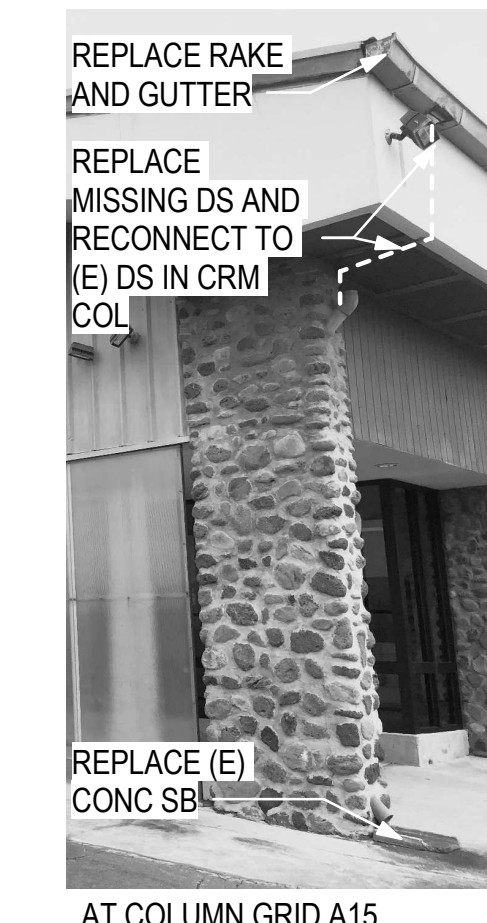
AT COLUMN GRID A15
